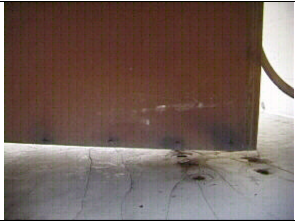
Damaged flooring under the bait station.
