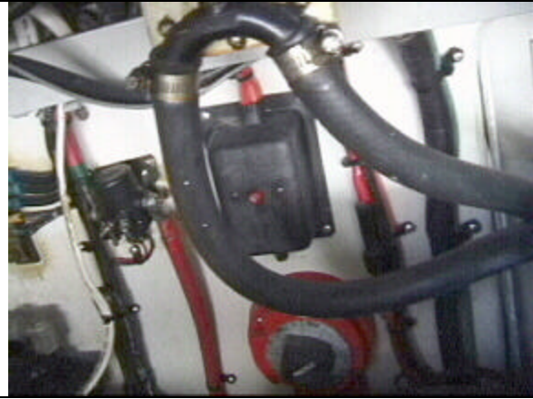
View of port side forward bulkhead in engine room. Note siphon break for generator, solenoid for starting generator, fuse box and battery selector.
